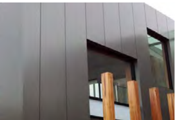
F11: ALUCOBOND CLADDING - SILVER METALLIC FINISH
