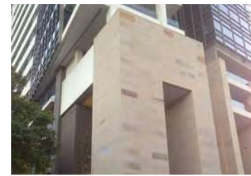
F1: SANDSTONE CLADDING
