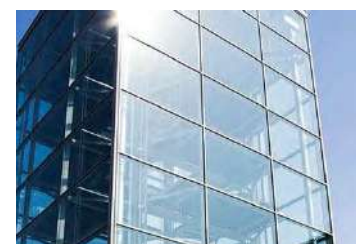
F13: CAR PARK FACADE
