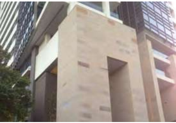
F1: SANDSTONE CLADDING
