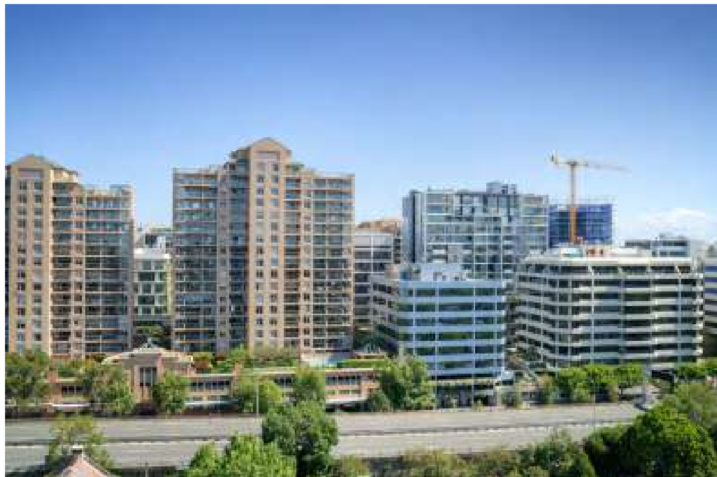
AERIAL VIEW FROM NORTH EAST - EXISTING
