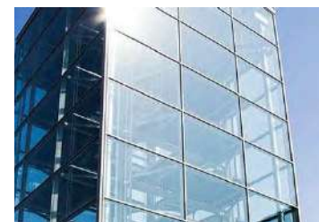
F13: CAR PARK FACADE
