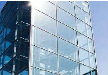
F13: CAR PARK FACADE
