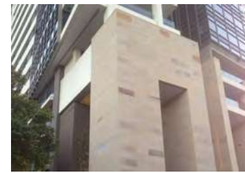
F1: SANDSTONE CLADDING
