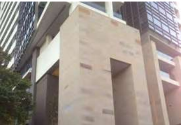
F1: SANDSTONE CLADDING
