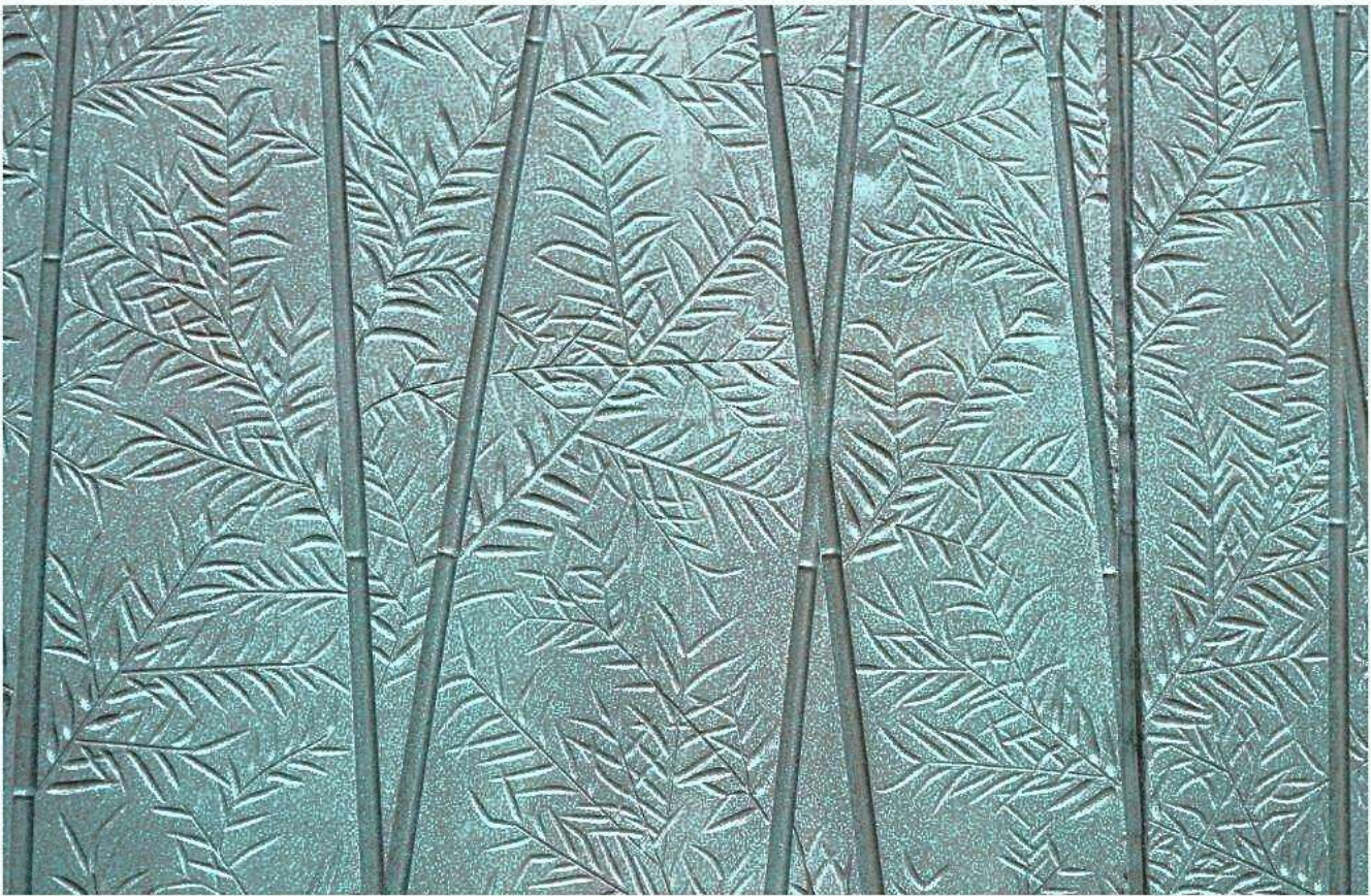
STENCILED PRE-CAST CONCRETE PANELS
