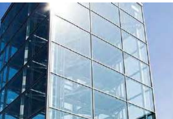
F13: CAR PARK FACADE
